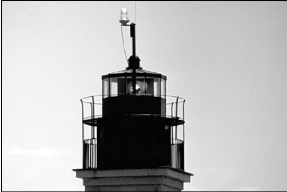
The lantern at Beavertail Lighthouse. In 1991 the fourth order Fresnel lens was removed from the lantern. It was replaced with a DCB-24 search light.
