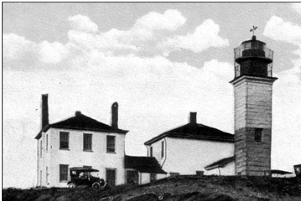
Beavertail Lighthouse in the 1920s. In 1898, a brick addition, an assistant keeper's dwelling, was built on the left side of the 1856 Beavertail Lighthouse keeper's dwelling and granite light tower.
