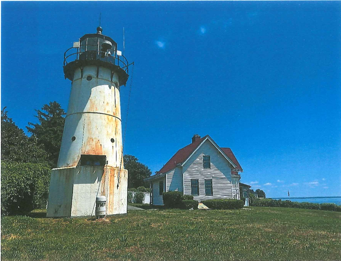
Photo 1. WARWICK NECK LIGHTHOUSE AND KEEPER'S QUARTERS, looking north.
