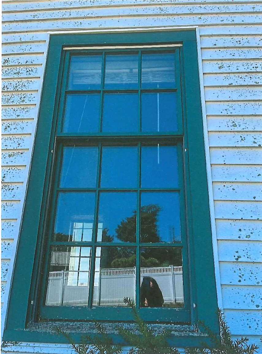
Photo 9. WARWICK NECK KEEPER'S QUARTERS, replacement window, typical.
