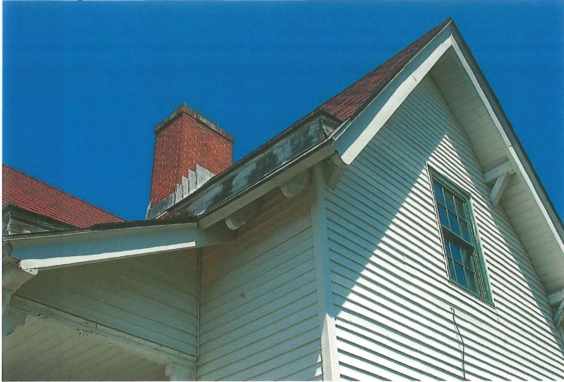
Photo 10. WARWICK NECK KEEPER'S QUARTERS, eave detail.
