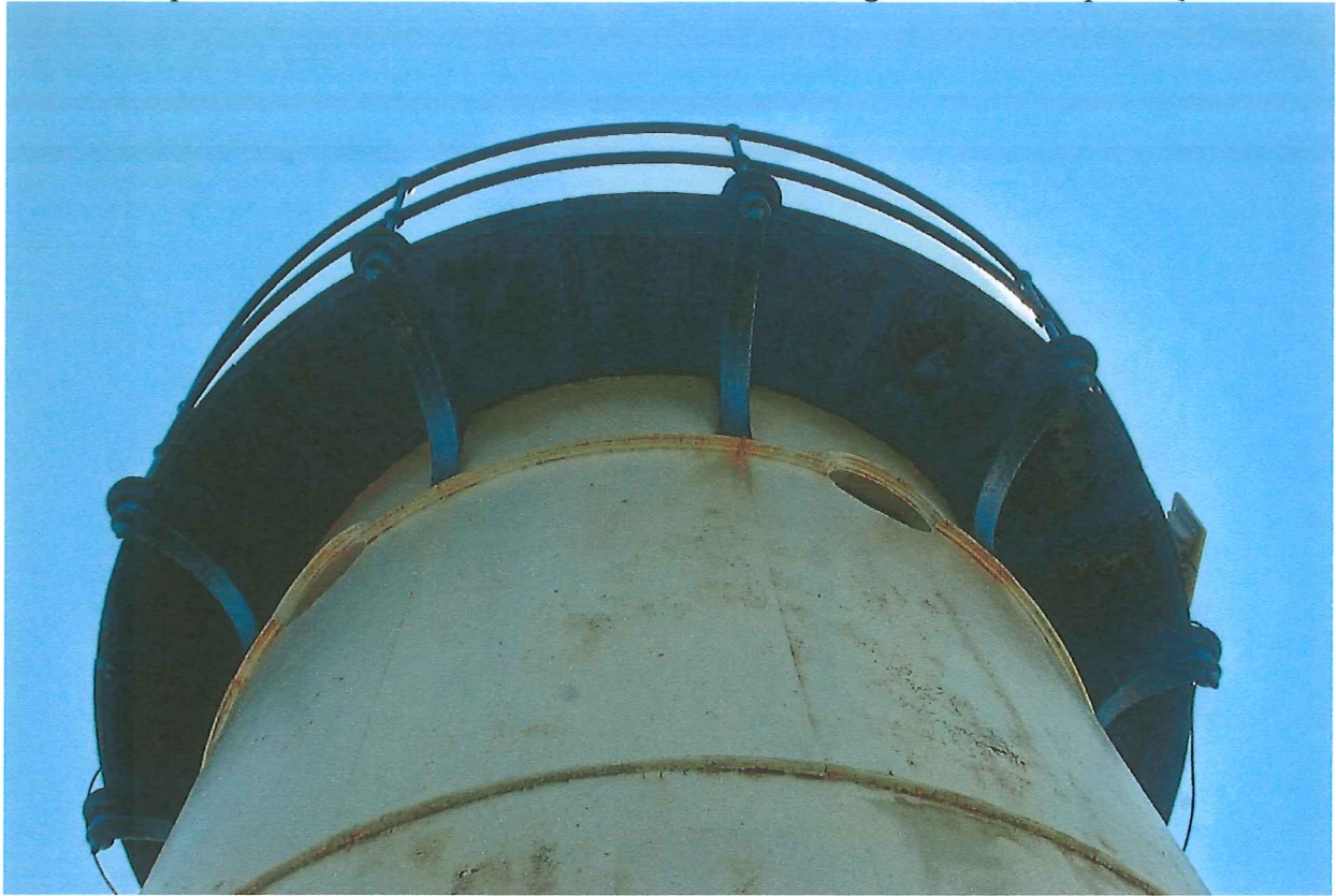
Photo 14. WARWICK NECK LIGHTHOUSE, gallery and bracket detail.
