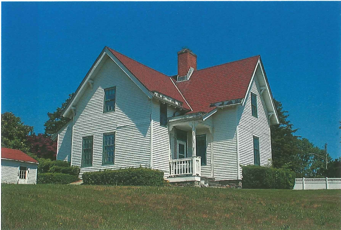
Photo 3. WARWICK NECK KEEPER'S QUARTERS, looking northwest. Note, damaged vinyl siding should be repaired to prevent damage.
