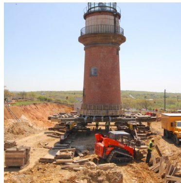
Gay Head Tower in the process of moving
