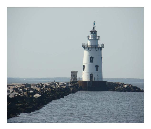
Saybrook Breakwater Light was one of the first of a number of cylindrical cast-iron lighthouses built between 1880 and 1920. The 49-foot tower is supported by a cast-iron concrete-filled caisson, a water tight chamber used in underwater construction work. The caisson was assembled on land nearby, taken by barge to the site and sunk into 17 feet of water. At the time, this method of construction was considered very common and cost effective.
