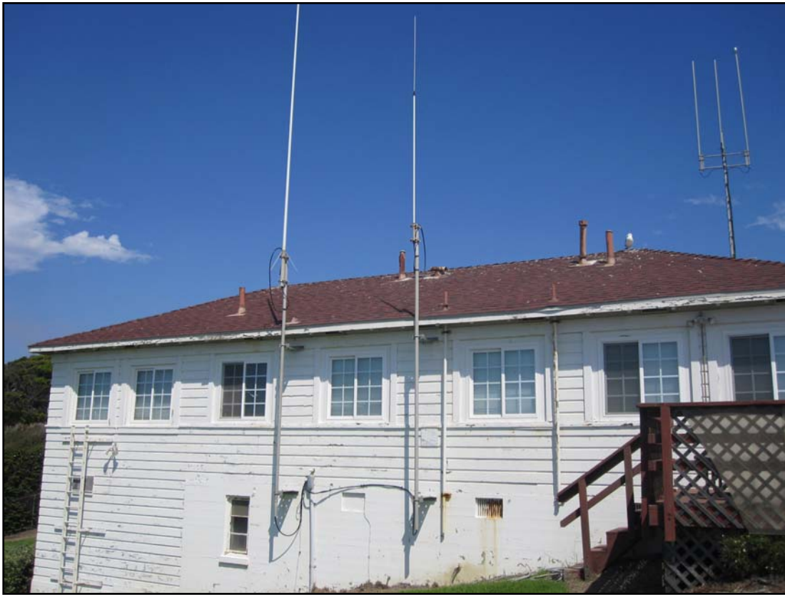
REAR VIEW OF GUEST QUARTERS FACING NORTH
