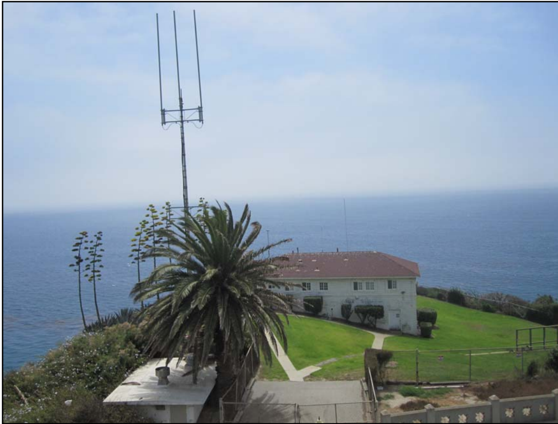
SEAWARD PARCEL - ELECTRONICS SHACK & ANTENNA, GUEST QUARTERS
