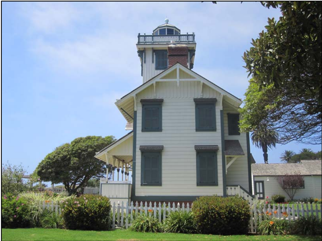
SIDE VIEW LOOKING WEST
