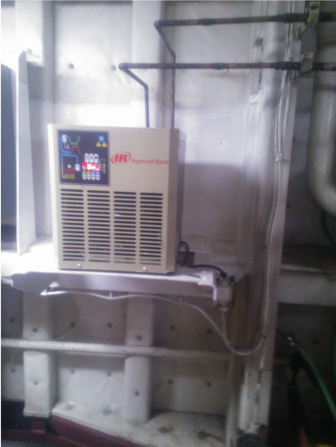
FIGURE 1. NEW AIR DRYER INSTALLED FRONT VIEW
